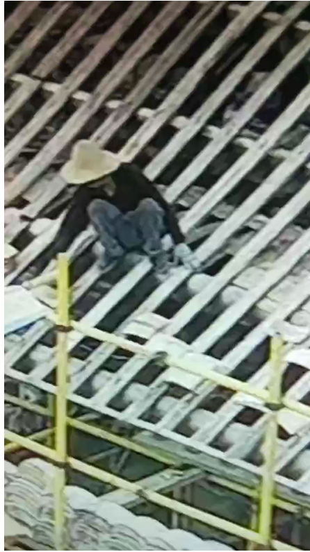
Worker removing the old roof.
